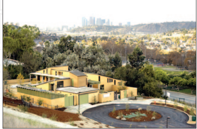
The Audubon Education Center in Debs Park, Los Angeles, won city approval to go "off the sewer grid" so it could capture, treat, and re-use wastewater with an AdvanTex Textile Treatment System (visible inside the traffic circle at the Center's entry). Pumps are solar-powered and effluent is disinfected and re-used for irrigation. This facility earned the first-ever Platinum LEED rating issued by the Green Building Council.
