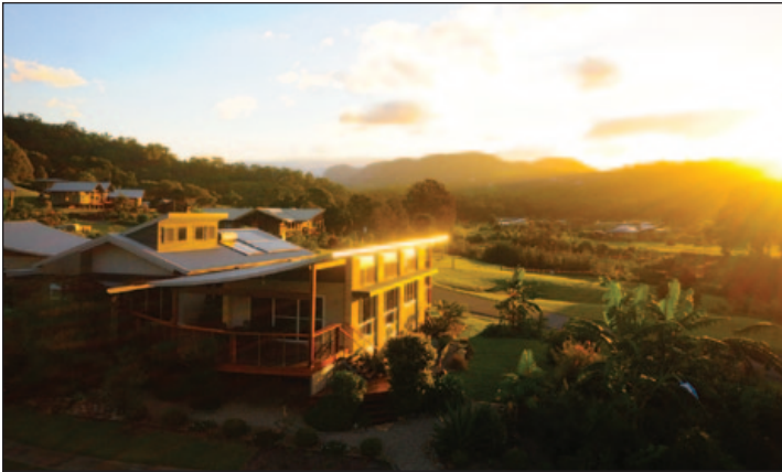
The EcoVillage at Currumbin, along the Gold Coast of Australia, uses AdvanTex® Textile Treatment Systems coupled with physical barrier micro-filtration, UV irradiation, and chlorine disinfection to produce water for non-potable uses that meets and exceeds Queensland EPA guidelines for Class A+ recycled water. The EcoVillage has won numerous international awards, including "World's Best Environmental Development."
