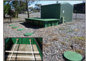
Greywater is cleaned for re-use with an AdvanTex Textile Filter, manufactured by Orenco.
